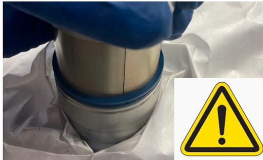
**#10** **Very important**.....make sure the dust wiper is level (squared up) with seal bore. Using the seal driver and with a twisting motion and push dustwiper into place. After dust wiper is seated you can also slide seal driver down a couple of times to make sure it's in place.
